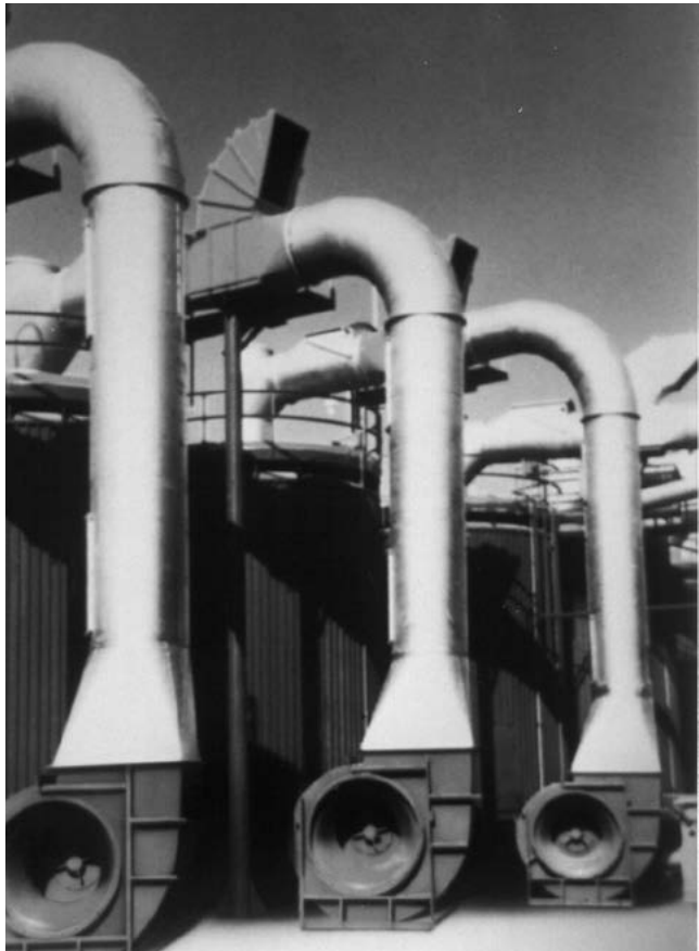
Figure 6. Well-designed duct configuration
